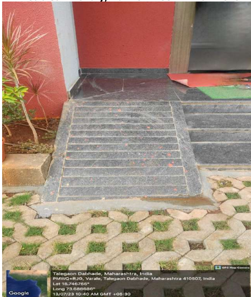
Ramp at the Entrance of the Building
