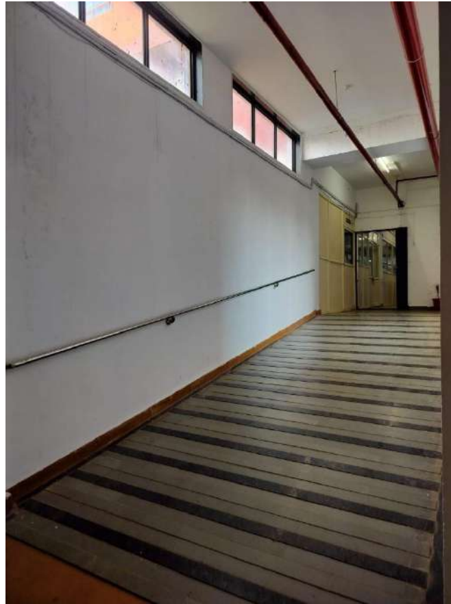
Ramp within the Building
